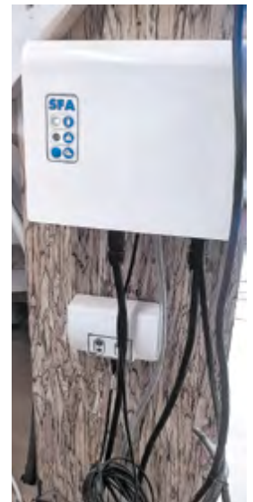
The control panel of the Sanicubic 1 has a visual and audible alarm system (including a 15’ wire).
